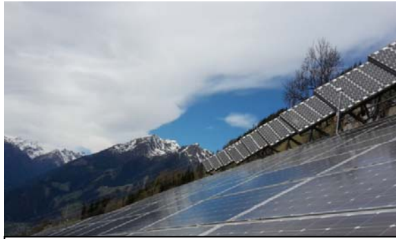
Caption 2: High-altitude radiation affects solar panels in the Andes, sand impairs output in Saudi Arabia, humidity causes problems in Tenerife and snow cover in the Austrian Alps reduces efficiency in winter. Different environmental conditions have an impact on solar energy output. PV solutions adapted to their environment are the basis for optimising system output and extending system lifetimes. © ENcome Energy Performance GmbH
